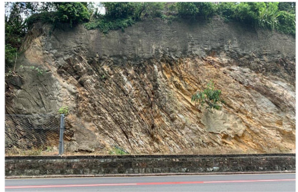
Fig 2. Tilted devonian metasedimentites of the Neranleigh-Fernvale Group at Adelaide Street, downtown Brisbane (Australia). These rocks, along with the Bunya phyllite, are one of the oldest rocks in Brisbane. The retaining wall at the bottom of the outcrop was built of 226-million-year-old volcanic tuff (Brisbane tuff) quarried in the city for years. (Photograph by J. Porras, 2024).
