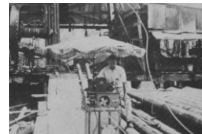
Equipment used in logging the first well in Maracaibo, Venezuela, in March 1929. The engineer plotted the log on chart paper, which was continuously driven by the wireline cable passing through two wheels coupled to the recorded mechanism. Source: Schlumberger.
