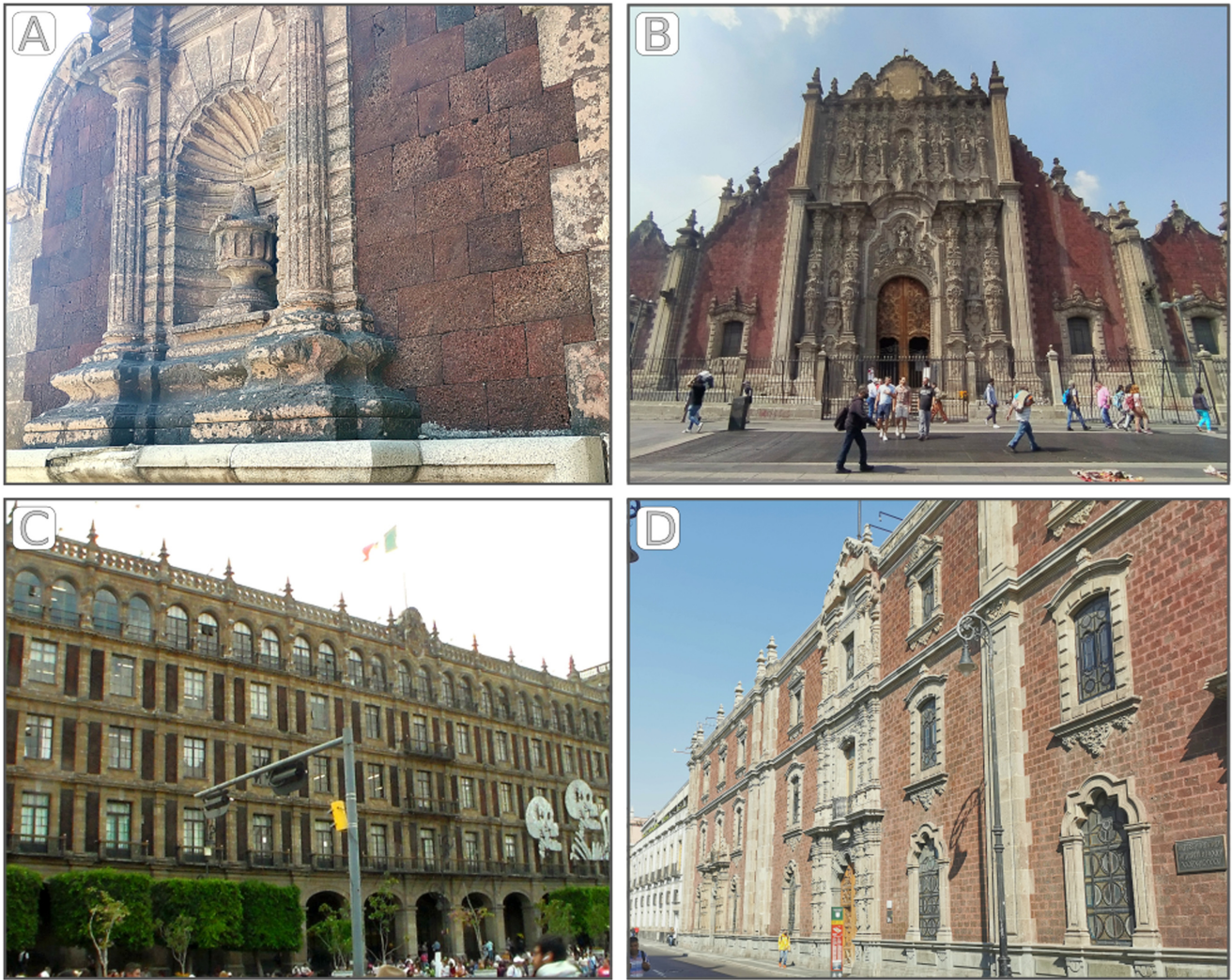
Figure 9. Prominent examples of the use of tezontle in monumental architecture in the Basin of Anáhuac, central Mexico: (A) Top of the Guadalupe Aqueduct, built between 1743 and 1751, made with reddish tezontle ashlars combined with gray tuff decoration. (B) Main façade of the Tabernacle of the Catedral Metropolitana (Mexico City Metropolitan Cathedral), built between 1749 and 1768. From the last phase of the Churrigueresque Baroque style, this monument is characterized by the stipite columns framed by walls with tezontle cladding. (C) Palacio de Gobierno (government building) of Mexico City. Its construction began in 1527, being the oldest building for which materials looted from previous Mexica temples were used. In spite of its overlapping of later construction stages, it preserves the Spanish (peninsular) Baroque style, with the particularity of interspersing the gray tuff fine decoration with reddish tezontle rough cladding. (D) South façade of the Colegio de San Ildefonso, former Jesuit college that is currently a science museum. Of baroque style, construction of this building began in 1583. Windows are highlighted with mixtilinear arches and decorated frames done with clear tuff; the delicate decoration is emphasized by contrasting it with the reddish tezontle façade cladding. Locations: (A) Alcaldía (borough) Gustavo A. Madero, Mexico City. (B), (C) and (D) Alcaldía Cuauhtémoc, Mexico City, within the “Historic Centre of Mexico City and Xochimilco” UNESCO World Heritage site (WHC, 2023).
