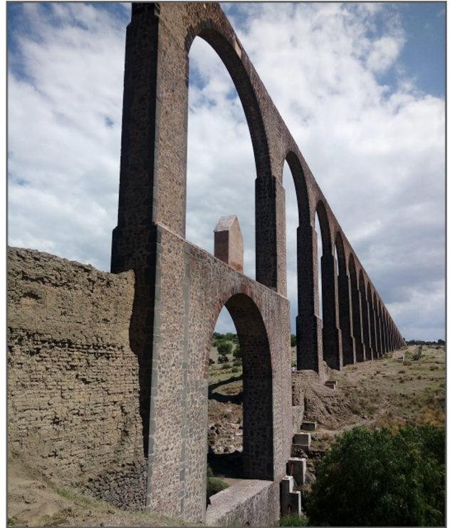
Figure 10. Acueducto del Padre Tembleque, registered in the UNESCO World Heritage List as “Aqueduct of Padre Tembleque Hydraulic System” (WHC, 2023). Built between 1555 and 1564, it crosses the Tepeyahualco ravine, extending between four municipalities: Axapusco and Otumba (State of Mexico), and Zempoala and Tlanalapa (Hidalgo). The central part of the bridges is built with finely carved tezontle masonry, including pilasters and the profiles of the voussoirs of the arches.
