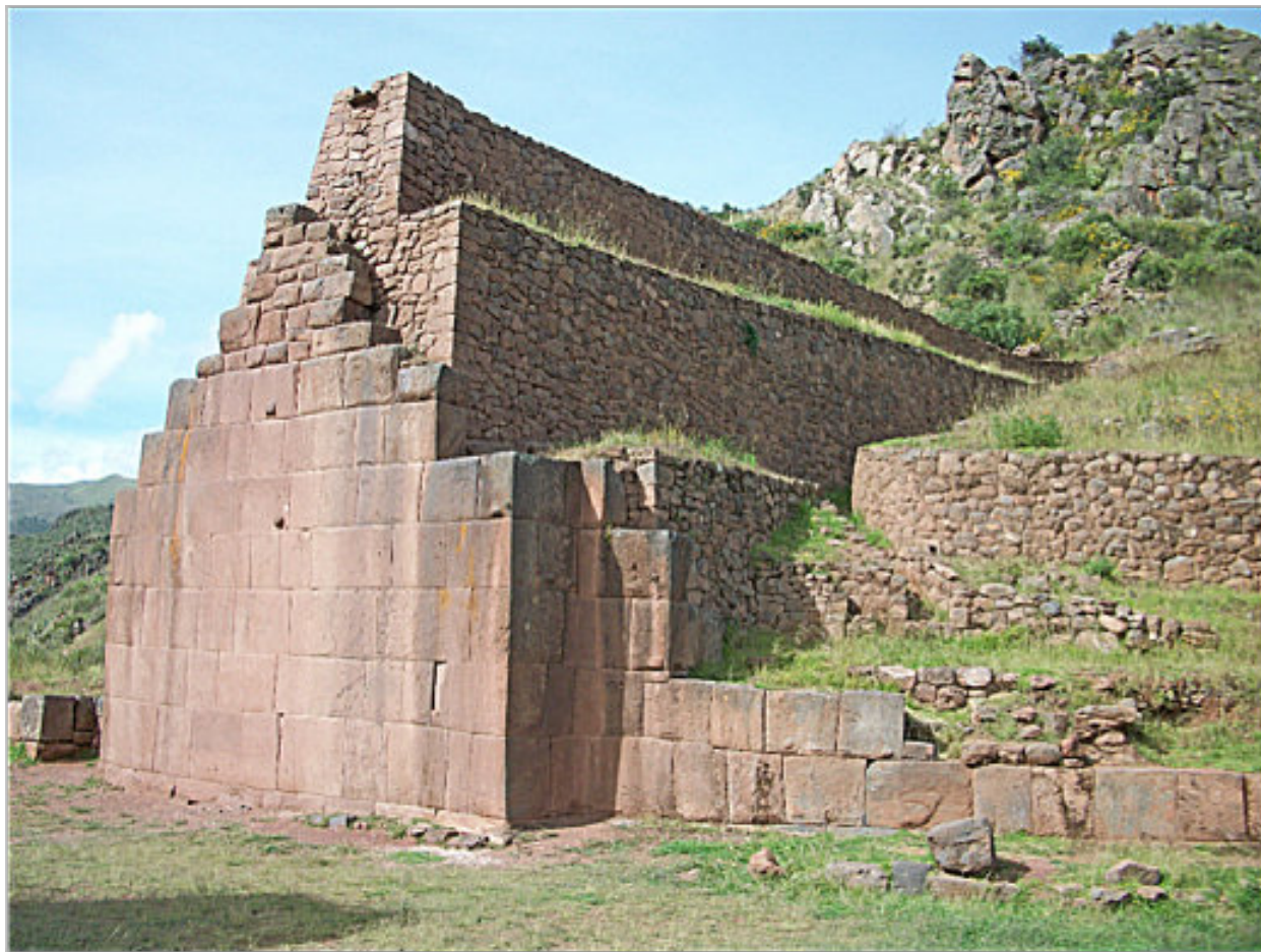
La Portada at Rumicolca. Note the veneer of Inca stonework over cruder Wari stonework. Photo courtesy of Renniksd, Wiki Commons.
