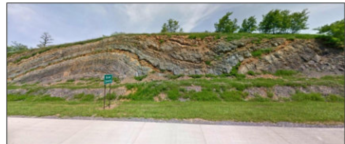
Fig 33. Street View north at anticline-syncline pair exposed in a roadcut, US-48 at the Grant County line, Virginia. © 2019 Google Street View.
